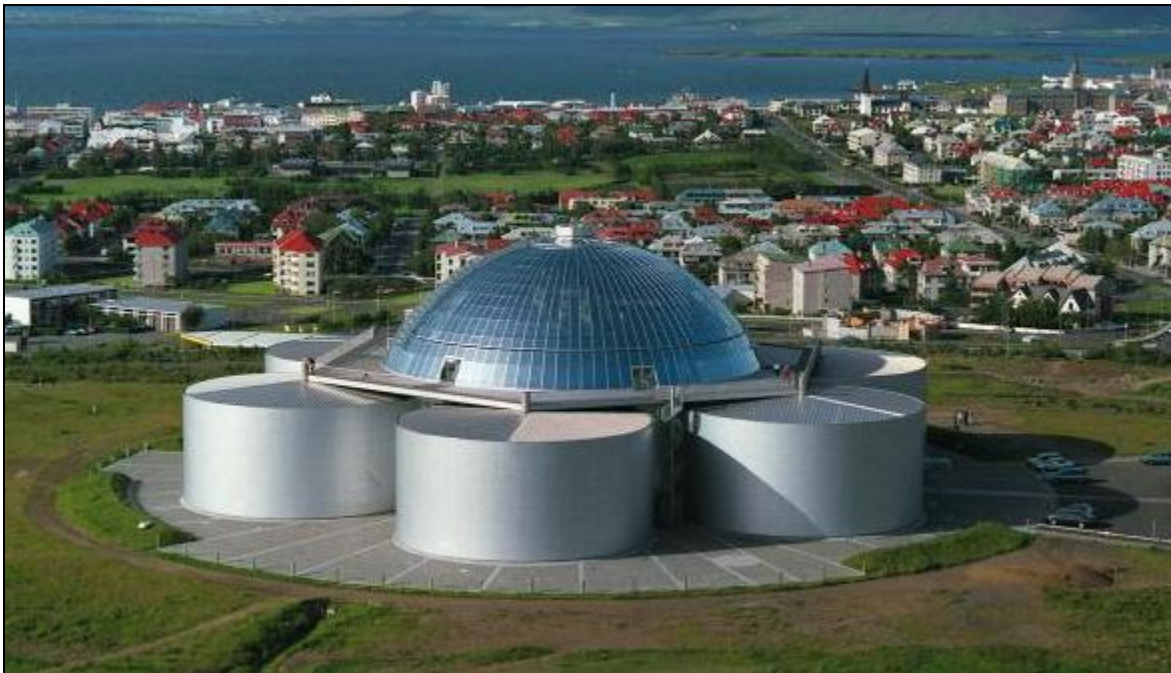
Figure 3 - The Pearl, Hot-water Tanks in Reykjavik
